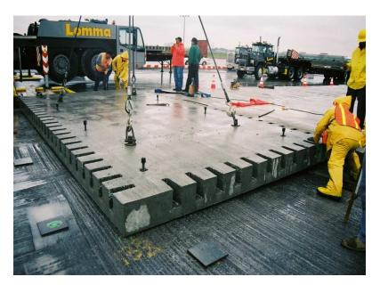
Figure 27. Precast full-depth slab replacement (courtesy Shiraz Tayabji).
