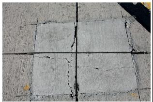
(c) Patching (high-severity) – Distress in patch has begun to spall and poses FOD potential.
