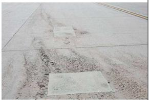
(c) Surface honeycombing (high-severity) – Large areas (greater than half the slab) in which the surface is open. Note patching is also present.
