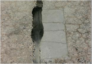
(b) Patching (medium severity) – Patch is intact, but cracked. Note that there is no current FOD potential.
