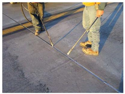
Figure 23. Joint resealing with silicone sealant (courtesy John Roberts, IGGA).
