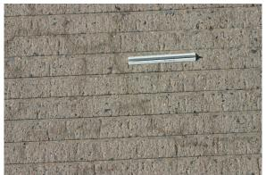
(b) Pattern cracking (low-severity) – Fine, tightly closed, cracking that is readily visible when dry. This cracking also has discoloration.
