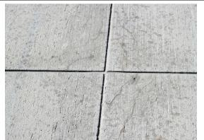
(a) Parallel cracking (low-severity) – Tightly closed cracking running parallel to joint and around corner. Discoloration (D) would be noted, as would staining (I).
