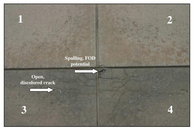
Figure 19. Example 5: cracking at slab corner with each corner numbered.
