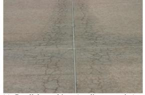
(c) Parallel cracking (medium-severity) – Open, parallel cracking at joints and around corner. Medium-severity perpendicular cracking is also present. Discoloration (D) would also be noted.
