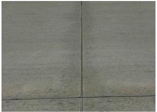
(c) Staining (locations 1 and 2) – Stained areas along joint and corners. Low-severity parallel cracking (G) at corner would also be noted.
