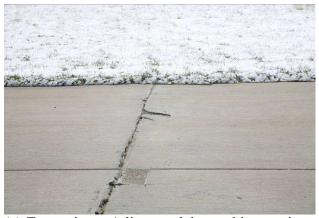
(c) Expansion - Adjacent slabs pushing against each other along joint caused this blow-up.
