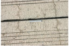
(b) Perpendicular cracking (low-severity) – Fine cracks perpendicular to a joint with discoloration (D).
