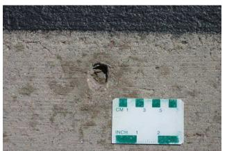
(b) Popout from clay ball – Deleterious materials that have disintegrated and left an opening on the surface of the pavement.
