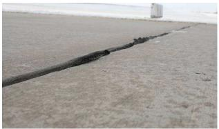
(b) Expansion – Expansion has closed the joint and caused sealant to bulge out.
