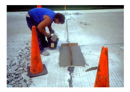
Figure 24. Partial-depth repair placement (courtesy Gary Mitchell, ACPA).
