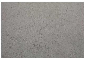
(a) Staining (location 3) – Lightly colored marks, blotches, or areas on a pavement not consistent with the normal pavement surface.
