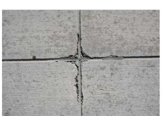
(a) Sliver spalling – Continuous areas are affected along joints or in corners that are greater than 1 ft in length.
