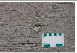
(a) Popout from aggregate – Reactive aggregates that have expanded near the surface and leave an opening on the surface.
