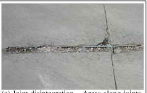
(a) Joint disintegration – Areas along joints are crumbling. Note that cracking is not parallel cracking.
