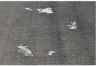
(c) Scaling – Interior areas have broken free with the potential for more scaling in cracked area.
