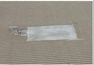
(a) Patching (low-severity) – The patch is present with no observable distress. Note that scaling (B) would also be recorded for this location.
