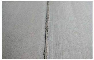
(b) Sliver spalling – Large, continuous areas are affected that are greater than 1 ft in length.
