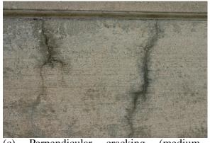
(c) Perpendicular cracking (mediumseverity) – Cracks are open and discoloration (D) is observed, but no FOD potential exists.
