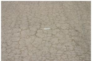
(c) Pattern cracking (medium-severity) – Well-defined pattern and some of the cracks have opened. Discoloration is also present.
