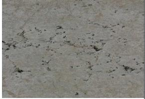
(b) Surface honeycombing (mediumseverity) –Isolated areas between  $1 yd^2$ and half the slab area where the surface is not closed.
