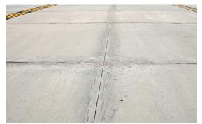
(b) Parallel cracking (medium-severity) – Open cracks running parallel to joint and around corner. In this case, exudate is present so Discoloration (D) would also be noted.
