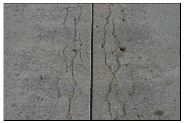
Figure 18. Example 4: opened cracking along joint.
