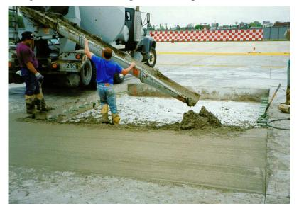
Figure 26. Conventional full-depth repair.
