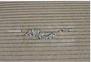
(b) Scaling – Small interior area has broken free and there is potential for more surface area loss in the cracked area.
