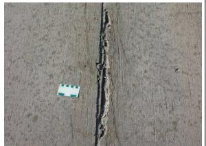
(b) Joint disintegration – Concrete along joint is crumbling/falling apart due to progression of parallel cracking. Note the visual difference between this distress and sliver spalling (no additional cracking).
