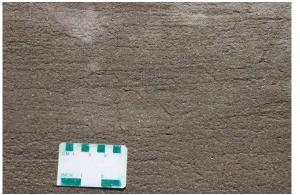
(a) Pattern cracking (low-severity) – Very fine pattern cracking that is barely visible and may only be seen when wetted.
