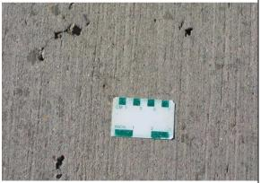
(a) Surface honeycombing (low-severity) – Small areas less than 1 yd<sup>2</sup> in size where minor openings in the surface resemble small popouts.
