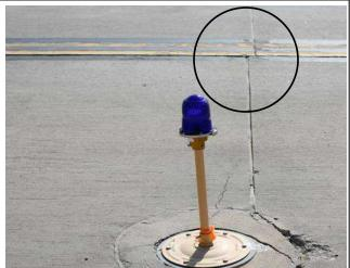
(a) Expansion – Shown in the circle is joint misalignment, which indicates an expansive movement, but the rater should confirm that the joints were originally aligned.
