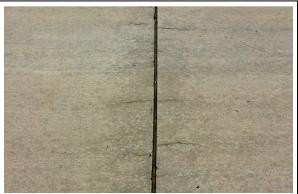
(a) Perpendicular cracking (low-severity) – Fine cracks perpendicular to a joint with discoloration (D).
